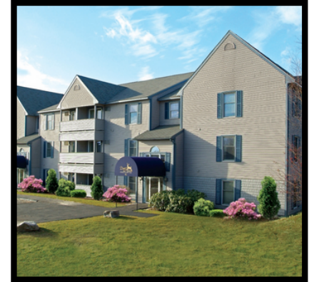
92 Eastern Avenue Manchester, NH
