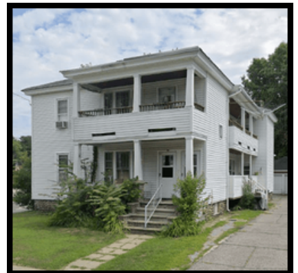
185 Calef Road Manchester, NH
